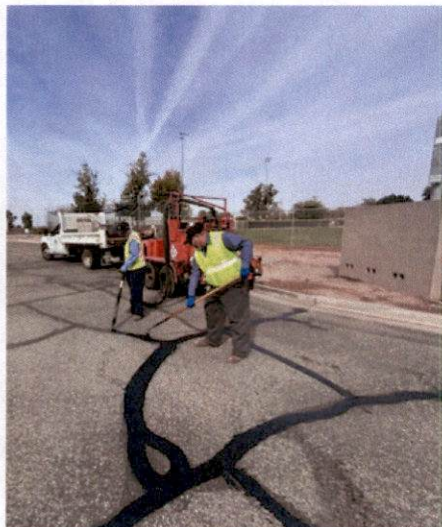
Crack Seal
