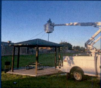
Bienestar Estates No.2 (700 6 th Dr.) Light was not working, new LED light was installed
