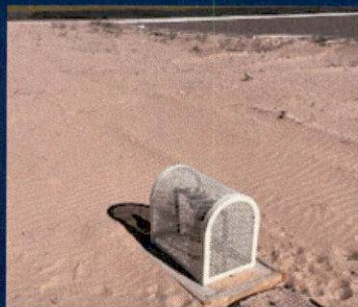
East Community Park (4005 Co. 24 th St.) New backflow cage was installed.
