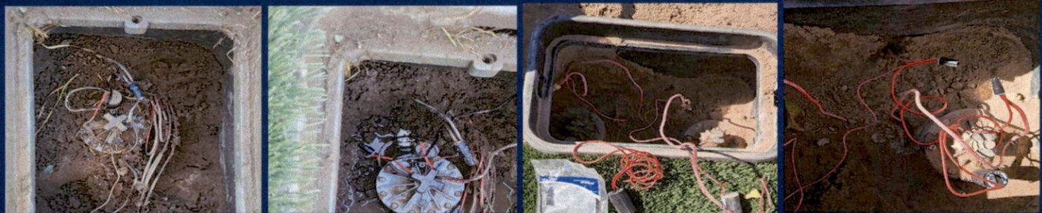
Rancho San Luis Unit1 (228 E Juarez St.) Repaired bad irrigation valve
